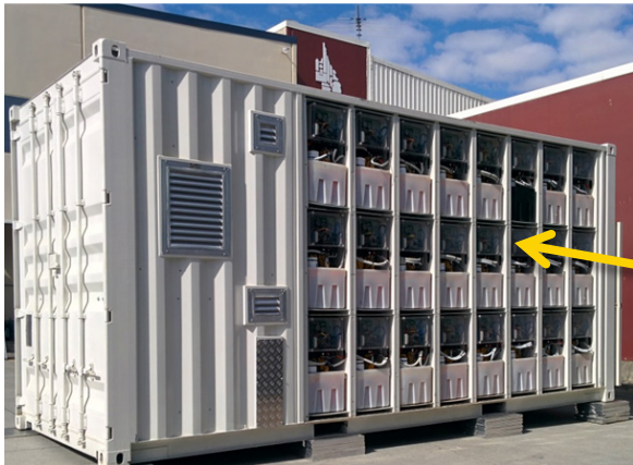
Figure 1. The Redflow large scale battery system (LSB)
